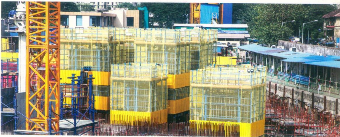
With jump form technology, the cycle time can be reduced from 12 days to seven days for core walls of two towers on an average, or sometimes even less.
